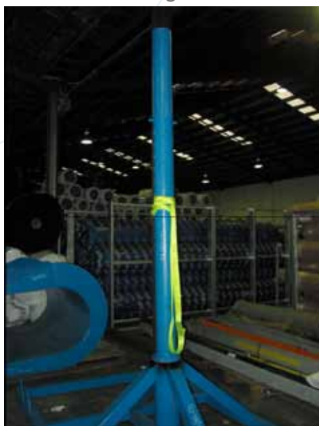
FEEDER HOPPER COLUMN AND SUPPORT POST
